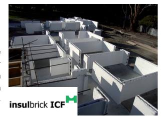
This project uses Insulbrick ICF 220 and 240 for all internal (200) and external (240) wall applications. This eliminated the need for timber framing altogether, as the walls are able to support a concrete roof on their own. The Owner / Builder of this project have installed the walls themselves, but did take advantage of one of the support packages which included bracing equipment/ block styrene cutting equipment plus experienced on site installers.
