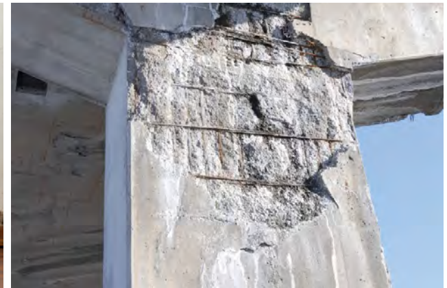
REBAR CORROSION
