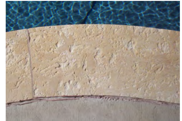
Unsealed travertine salt-water pool coping 5 months after installation.
