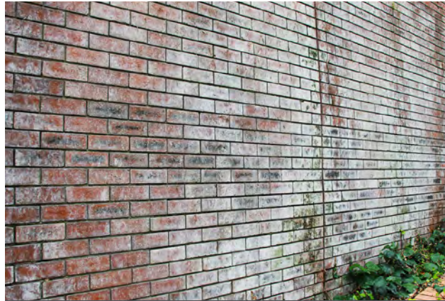
EFFLORESCENCE
