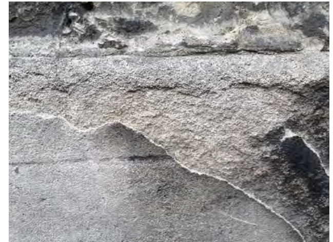
Delamination caused by freeze-thaw spalling.
