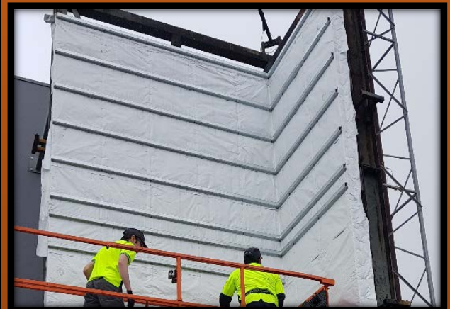
Steel top hats being installed
